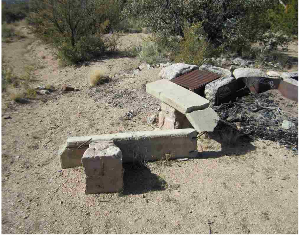
Figure 4. Historic concrete broken bench used for testing samples.
